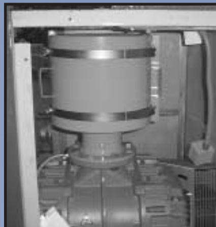
Lateral Access "LQB" Silencer Filter within a Compact Blower Enclosure
